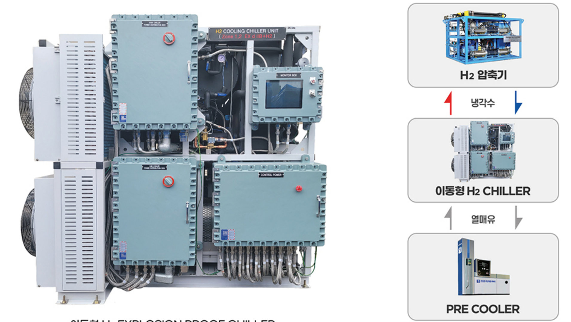
이동형 H 2 EXPLOSION PROOF CHILLER (Zone 1,2 EX d IIB+H 2 )
